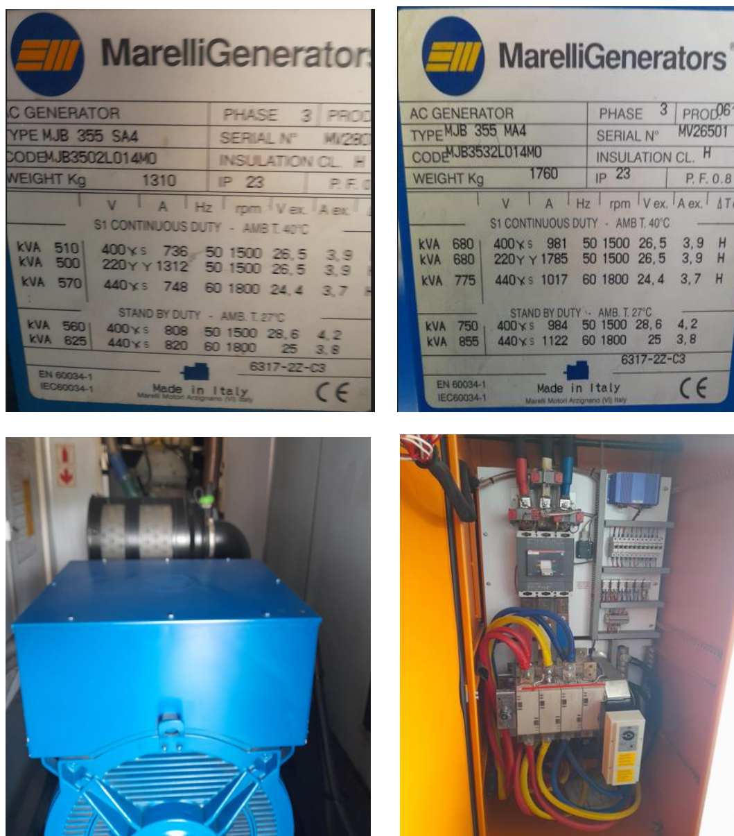
Figure 3-6: EAL Admin Building Diesel Generator Specification
