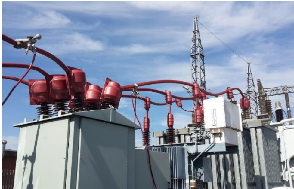
Figure 11: MV transformer bay with clamp and conductor insulation covers
