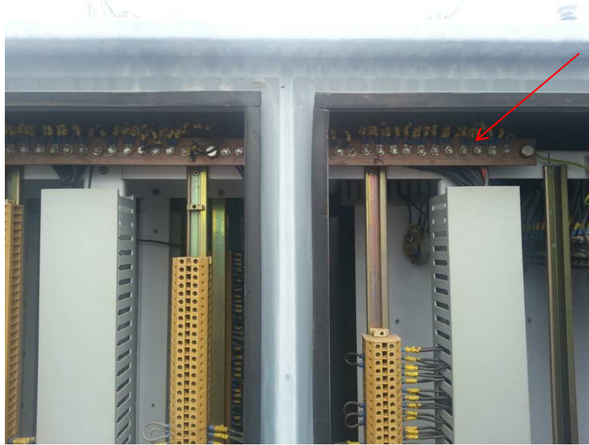
Figure 1: Properly earthed spare cable cores in yard JB
