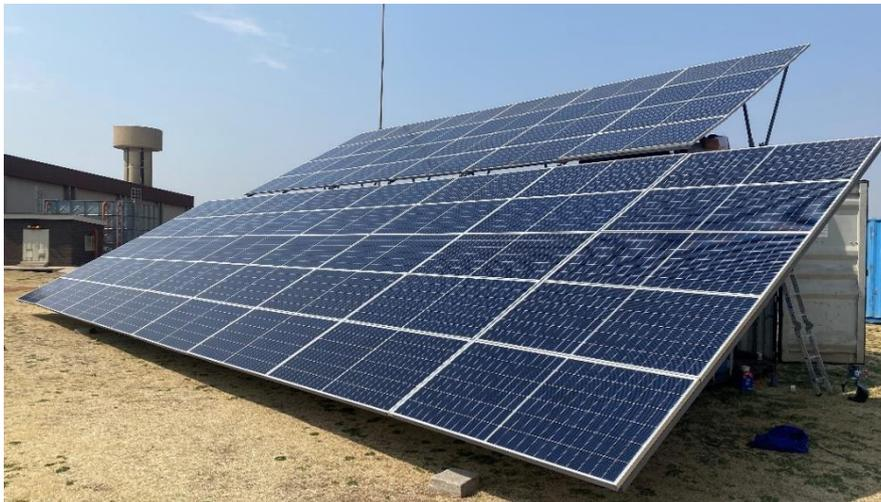
**Figure 1: Containerised Microgrid Solar Photovoltaic Generator and Battery Energy Storage System**
