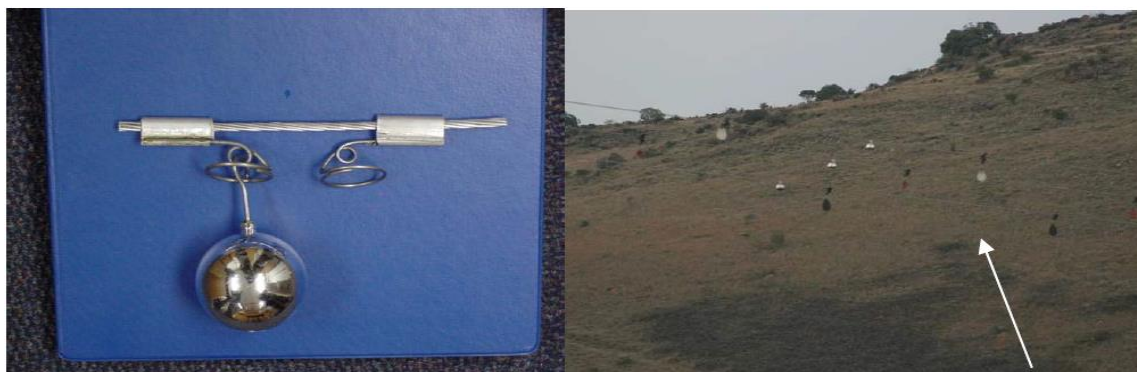
Figure 5: A Reflective Bird Diverter (left) installed on a line with conventional bird flappers (right)
