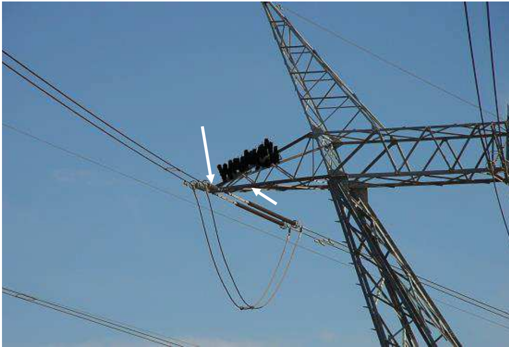
Figure 3-4: Picture of incorrect fitting leaving the landing plates, and the inside of crossarm, exposed.
