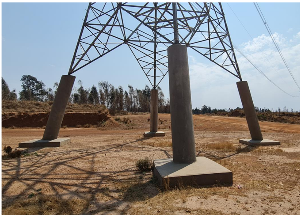
Figure C2: Example of a raised foundation columns on a tower
