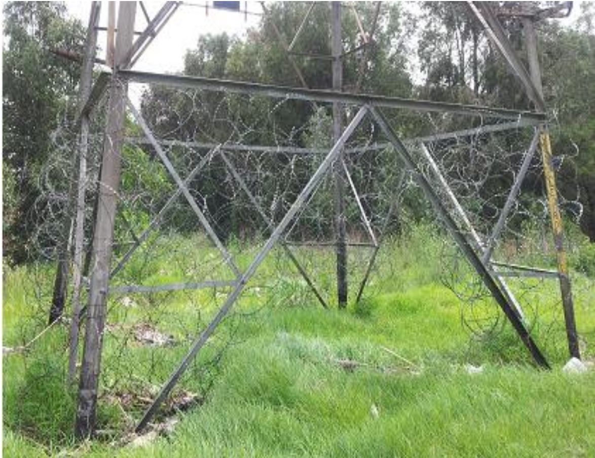
Figure F1: Example of a razor flap wrap around the tower members
