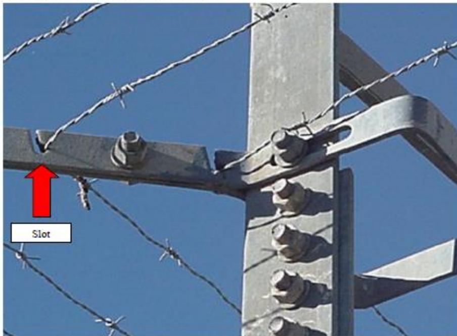
Insert 2: Barbed wire captured by vertical slots
