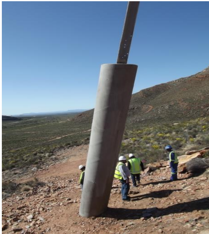
Figure C1: Example of a raised foundation column
