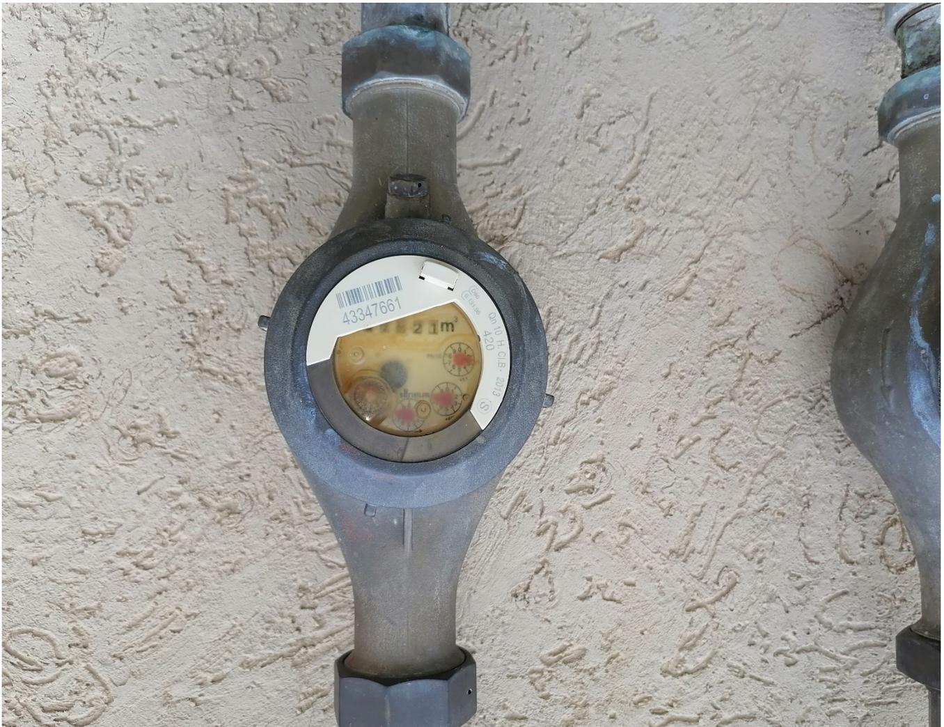
**Brass Water Flow Meter's Specifications.**1(a) Make: **SENSUS**(b) QP **10 H**(c) PN **16 kPa**(d)  $\Delta P$  **100kPa**(e) Face to face length =**320mm**(f) Water Flow Meter Port sizes on both sides **G 1 ½" (inch)** or **DN 40mm**(g) Compression fitting size **G1 ½" (inch)**(h) The quantity of water flow meters to be purchase, **Qty x 3****CONTROLLED DISCLOSURE**
