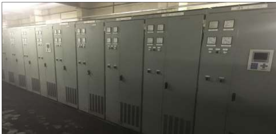
Figure 3-6: Control Panels for Existing Precipitator Rectifier Transformers
