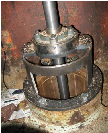
Figure 11.2.3: 2007 Guide vane middle bush boring
