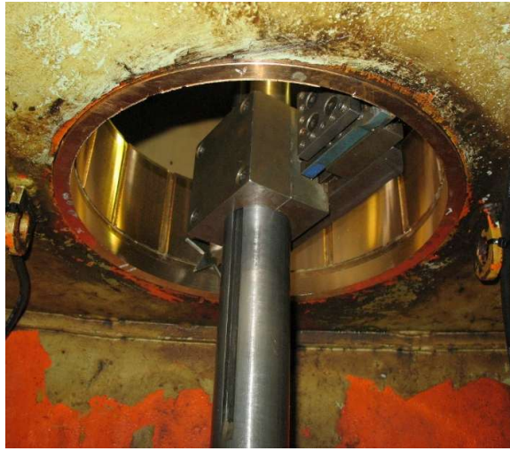
Figure 11.2.2: 2007 Guide vane top bush boring
