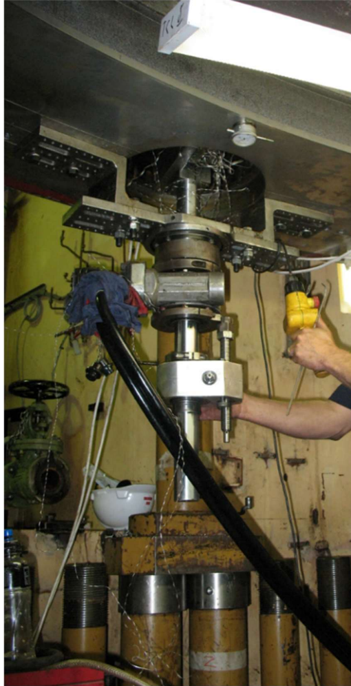
Figure 11.1.1: Guide vane bush casing repairs
