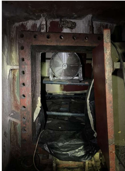
Figure 11.4.2: Draft tube mandoor with sealing surfaces on flange
