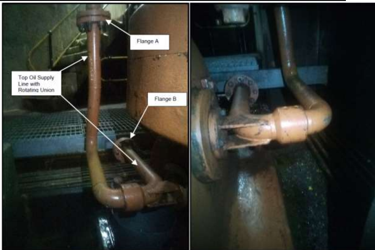
Figure 1: Existing Oil Supply Pipe Rotating Union
