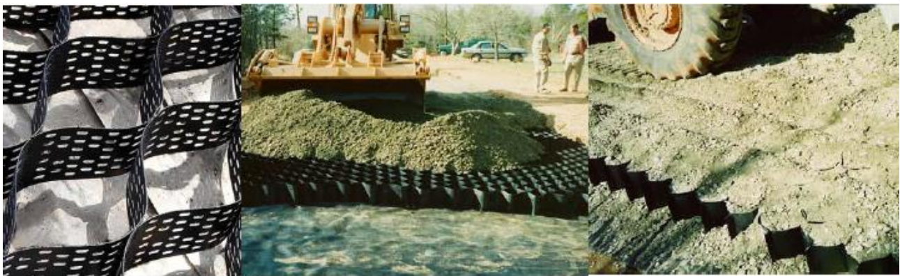
Figure F.9: Increasing load bearing capacity using a cellular confinement system (Sources: ElMich.com and Geoproducts.org)
