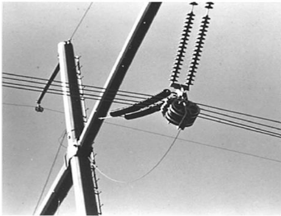
a) Application of traveler ground
