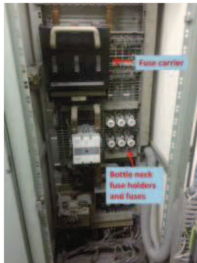
Figure 9: HV control panel
